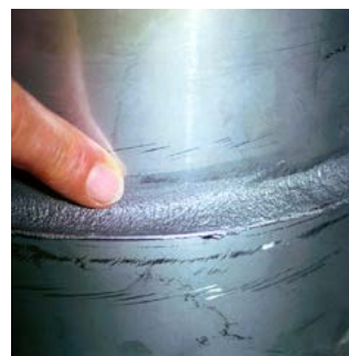
Pyro-Putty® 2400 seals high temp ducting.
