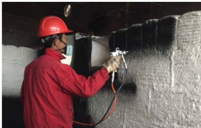
HiE-Coat™ 840-C applied to ceramic fiber module.
