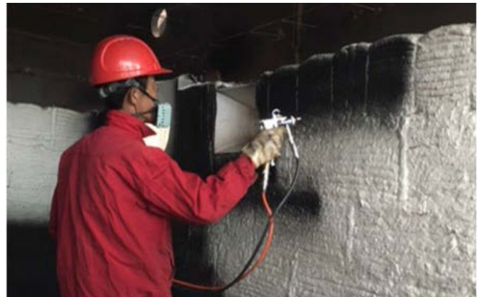
HiE-Coat™ 840-C applied to ceramic fiber module.
