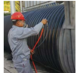
HiE-Coat™ 840-M coats industrial heat exchanger.
