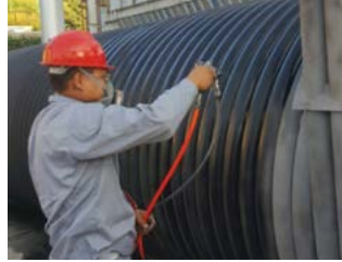
HiE-Coat™ 840-M coats industrial heat exchanger.
