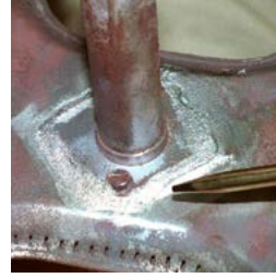
Pyro-Putty® 653 seals corroded burner manifold.
