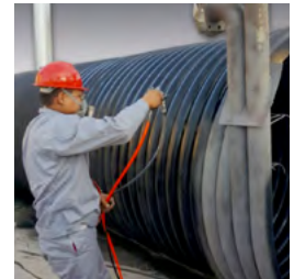
HiE-Coat™ 840-M coats industrial heat exchanger.
