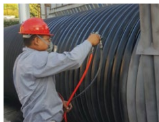
HiE-Coat™ 840-M coats industrial heat exchanger.
