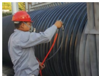
HiE-Coat™ 840-M coats industrial heat exchanger.
