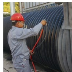
HiE-Coat™ 840-M coats industrial heat exchanger.
