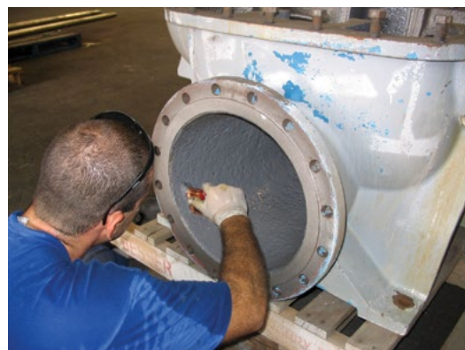
Corr-Paint™ CP2060 coats pump housing.
