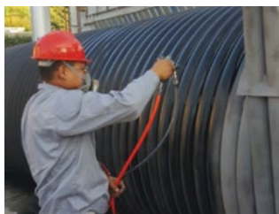
HiE-Coat™ 840-M coats industrial heat exchanger.
