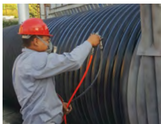
HiE-Coat™ 840-M coats industrial heat exchanger.
