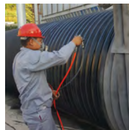
HiE-Coat™ 840-M coats industrial heat exchanger.
