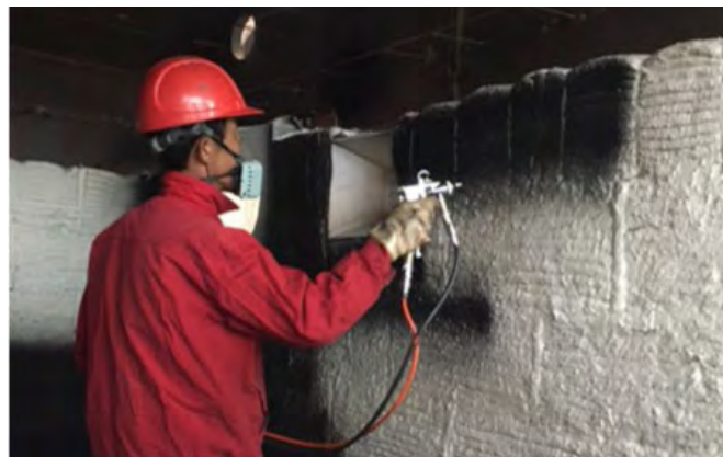
HiE-Coat™ 840-C applied to ceramic fiber module.
