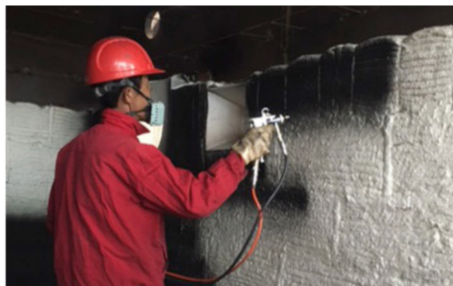
HiE-Coat™ 840-C applied to ceramic fiber module.
