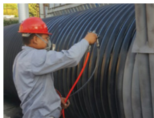
HiE-Coat™ 840-M coats industrial heat exchanger.
