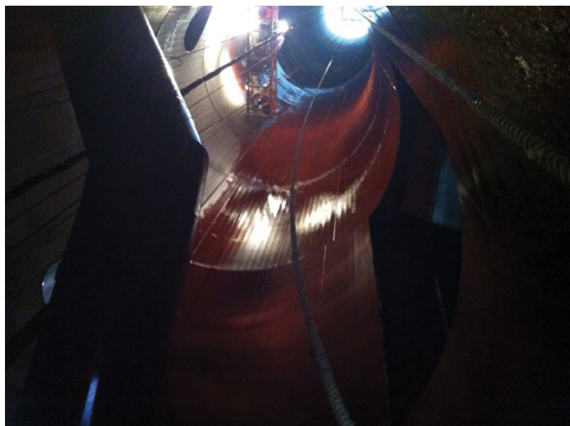
Corr-Paint™ CP2050-LF coats flare stack.
