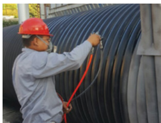
HiE-Coat™ 840-M coats industrial heat exchanger.
