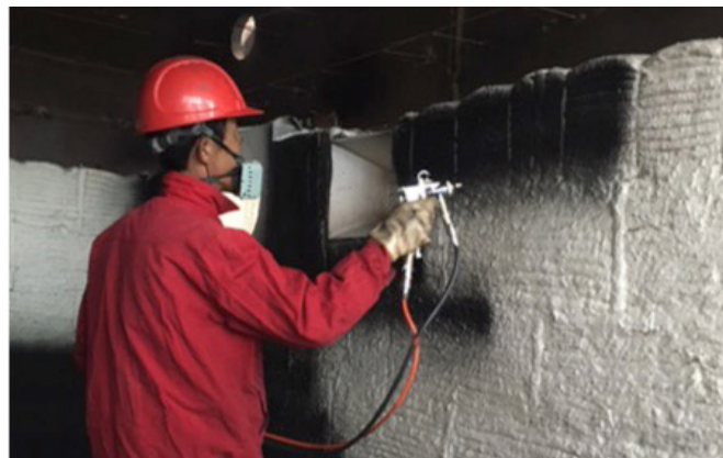
HiE-Coat™ 840-C applied to ceramic fiber module.
