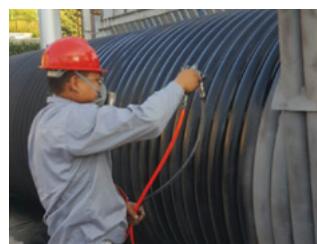
HiE-Coat™ 840-M coats industrial heat exchanger.
