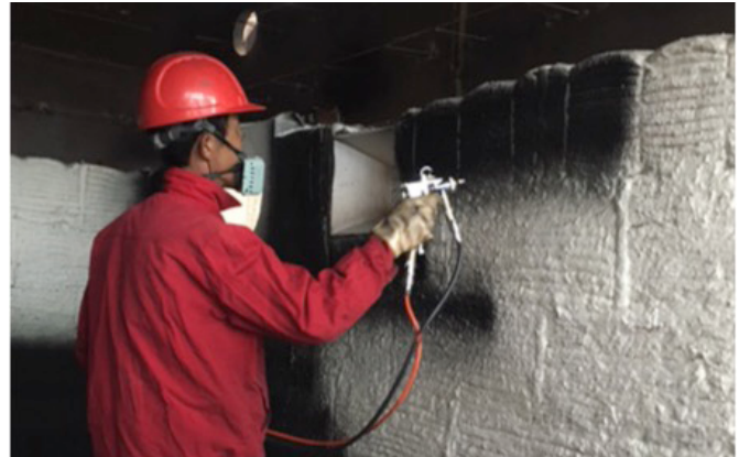
HiE-Coat™ 840-C applied to ceramic fiber module.
