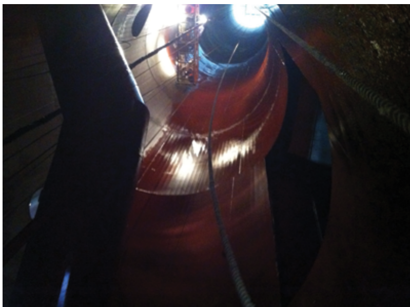
Corr-Paint™ CP2050-LF coats flare stack.
