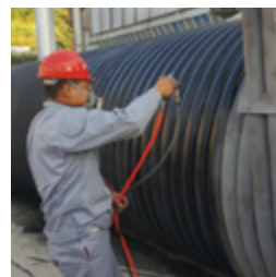
HiE-Coat™ 840-M coats industrial heat exchanger.
