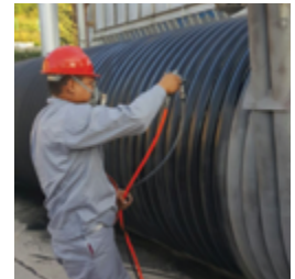
HiE-Coat™ 840-M coats industrial heat exchanger.
