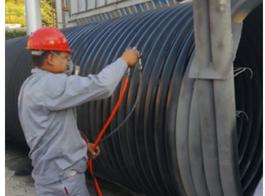
HiE-Coat™ 840-M coats industrial heat exchanger.
