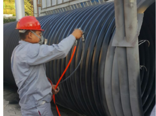
HiE-Coat™ 840-M coats industrial heat exchanger.
