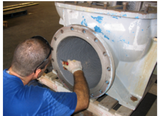
Corr-Paint™ CP2060 coats pump housing.
