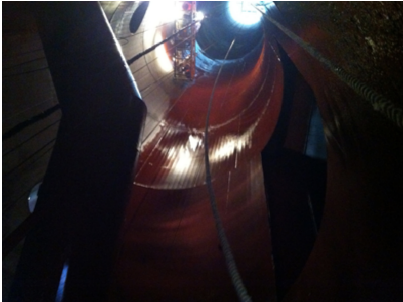
Corr-Paint™ CP2050-LF coats flare stack.
