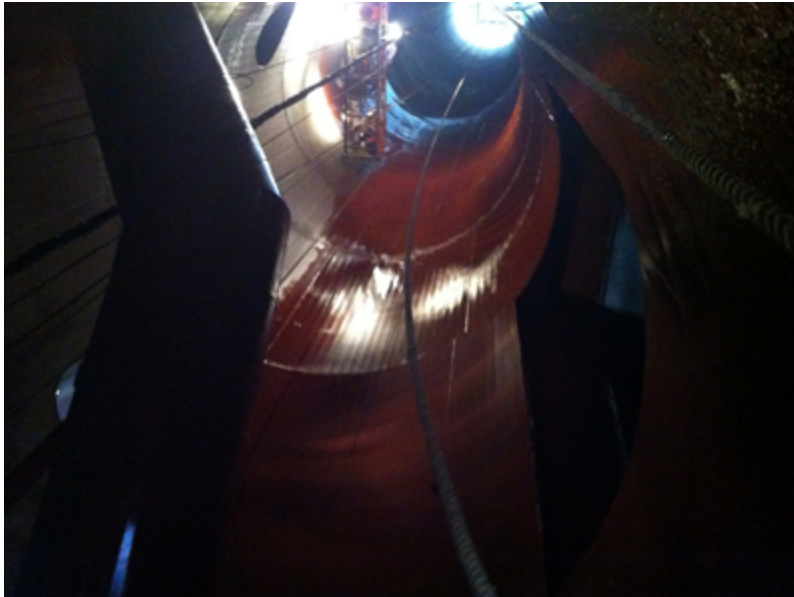
Corr-Paint™ CP2050-LF coats flare stack.
