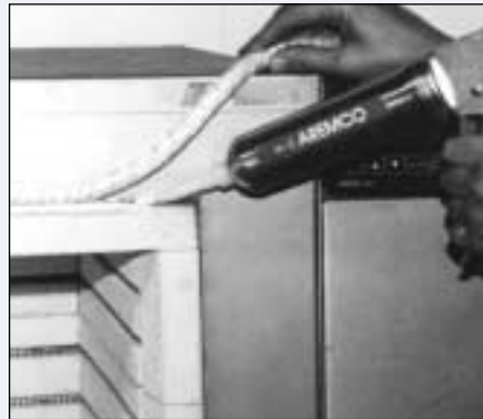
Pyro-Putty™ 600 bonds insulation rope.
